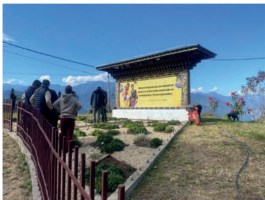
Picture 21.7 Construction of Royal portrait
