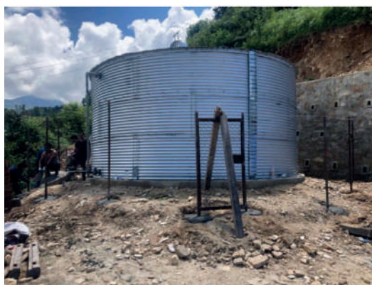
Picture 21.8 Construction of Mawongpa Water tank
