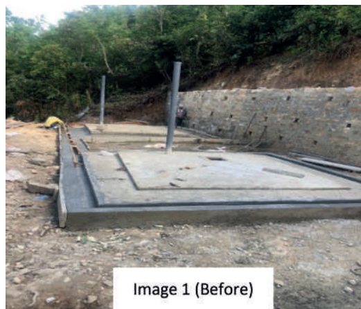
Picture 21.4 Construction of deep burial pit
