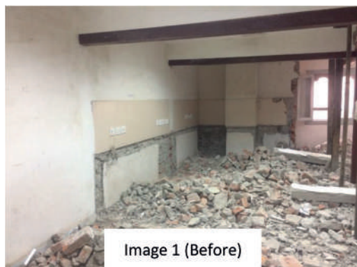
Picture 21.2 Remodification of Microbiology lab
