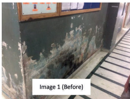
Picture 21.1 Renovation of ward
